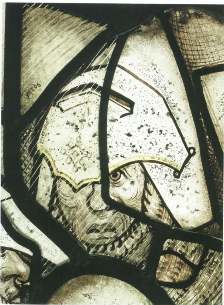
Fig. 5. Detail showing modern infills, installed by the York Glaziers Trust in 2008, Great East Window, York Minster (photo: author)
