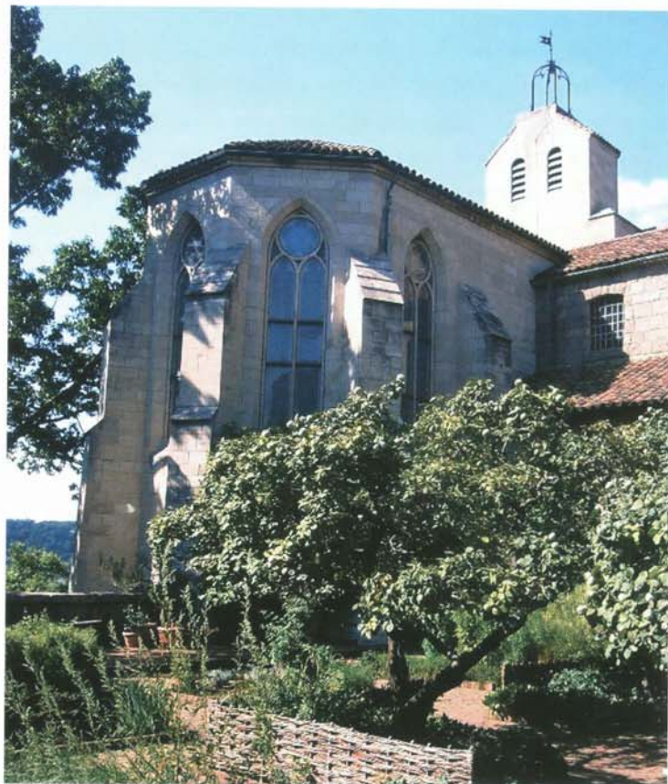
Fig. 6. Protective glazing with smooth panes, installed 2006, the Gothic Chapel, The Cloisters, New York (photo: author)
